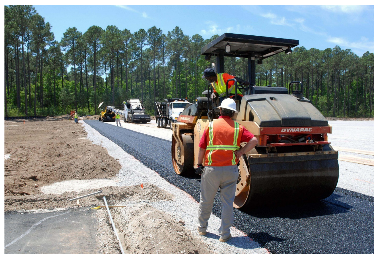
WMA is mixed and laid at lower temperatures, reducing emissions of GHG and air pollutants.
